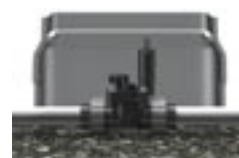
Coupling nuts are threaded onto the inlet and outlet of the valve
