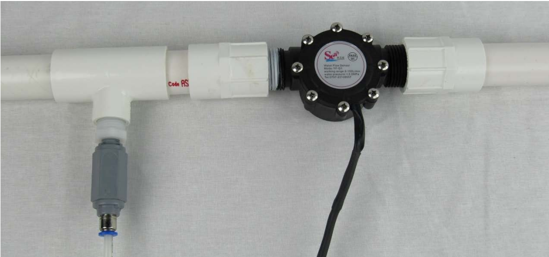
Installation in a straight section of mainline pipe
