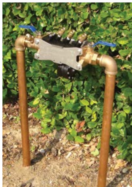
1" 375 Reduced Pressure Principle Assembly
